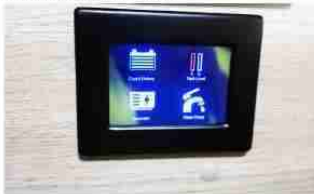
System Monitor Panel -Typical View
