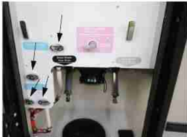
Waterline drain valves (Shown in the closed position turn valves to open). -Typical View
