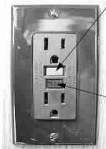
GFCI Outlet (Ground Fault Protector)
