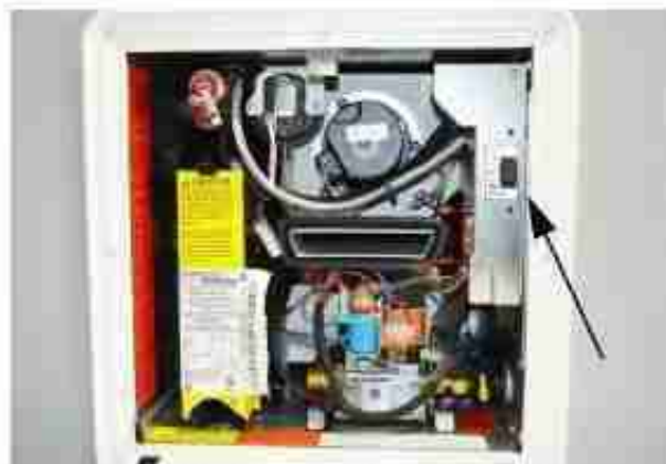
Water Heater Power Switch (Located behind water heater access panel on exterior of the motorhome)
